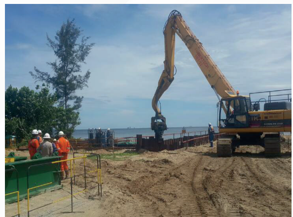
Installation of 24m lengths Sheet Piled Wall
