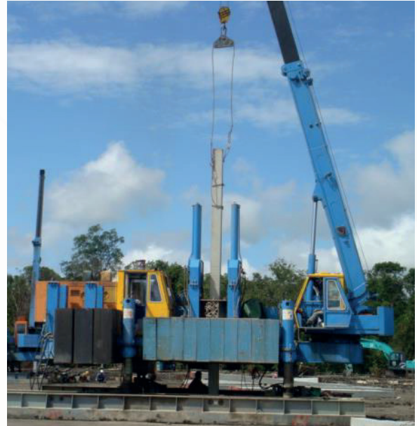
320 Tonne Injection Piling Rig
