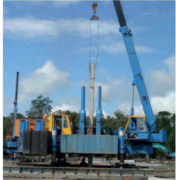
320 Tonne Injection Piling Rig
