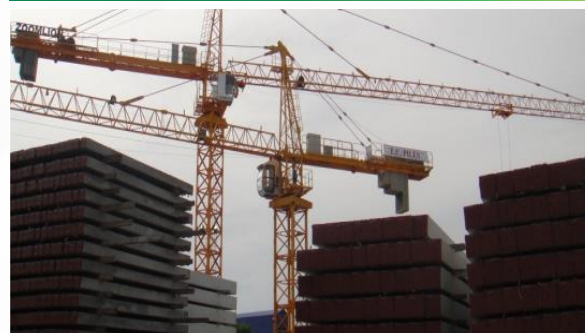
Stacking and distribution of TBT Piles by tower crane
