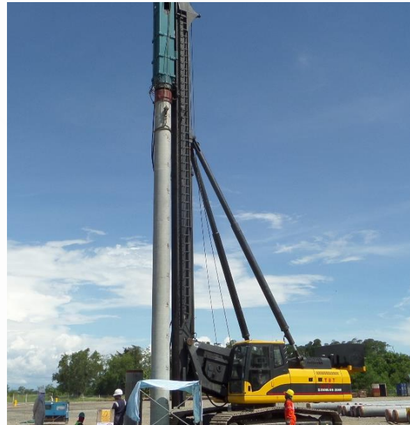
Installation of Prestressed Spun Piles
