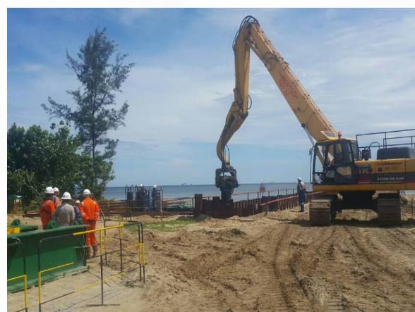
Excavator Mounted Vibro Hammer
