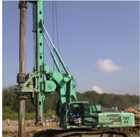
Rotary Drilling Rig
