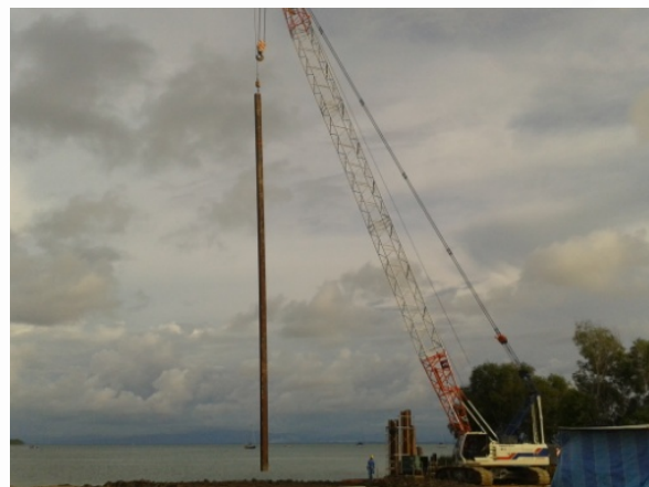
Installation of 24m Lengths Sheet Piled Wall
