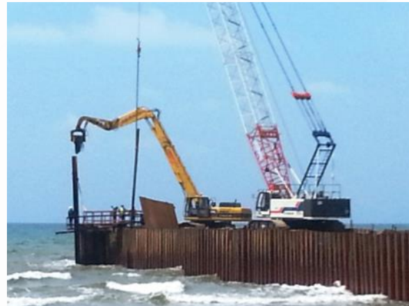
Cofferdam Sheet Piling Works Using Combination of Crawler Crane and Excavator Mounted Vibro Hammer
