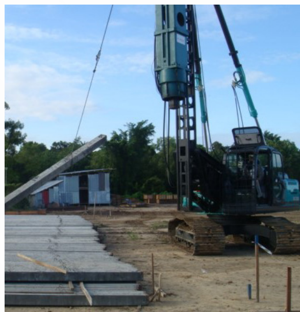
Installation of Precast R.C. Piles
