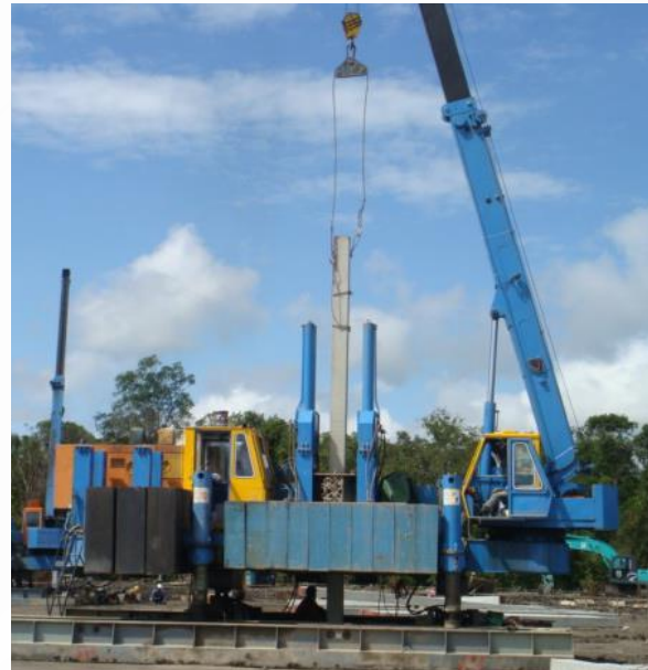
320 Tonne Injection Piling Rig
